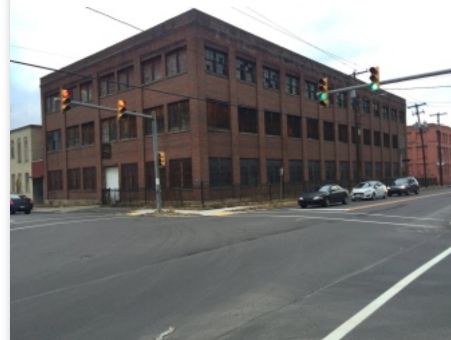
JIM LOCKWOOD / STAFF PHOTO Former Scranton Button Co. building on Cedar Avenue at Cherry Street in South Scranton.
